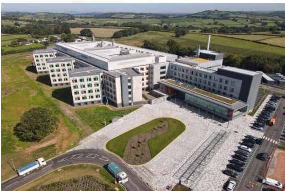
Modular built hospital- Grange University Hospital by Laing O'Rourke. Photograph by Paul Davies
